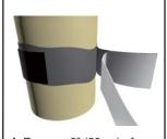
4. Remove 8" (20cm) of release backing and position exposed surface on cleaned and primered seam area. Expose 8" (20cm) sections at a time as you wrap the sleeve material around the entire circumference of the manhole.
