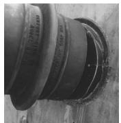
3. Place the Century-Line® Sleeve on the end cap. When field cutting non standard CS sleeve lengths, the sleeve and endcaps total length should be one-fourth (1/4") longer than the thickness of the wall. Cut with a hand or power saw. Note: To insure minimum water migration, center the water stop in wall by cutting equal lengths
