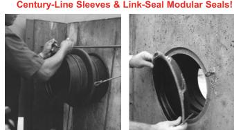
5. For additional stability, it's necessary to secure the sleeve with wire to the rebar. Insert the other end cap firmly, check that second end cap is positioned correctly, confirm sleeve length and close the
